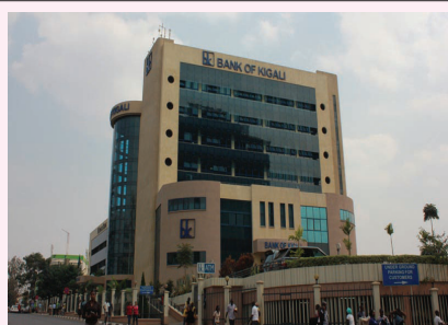
(a) Bank of Kigali
